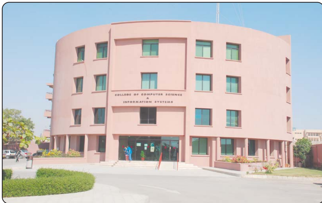
A View of IT Building
